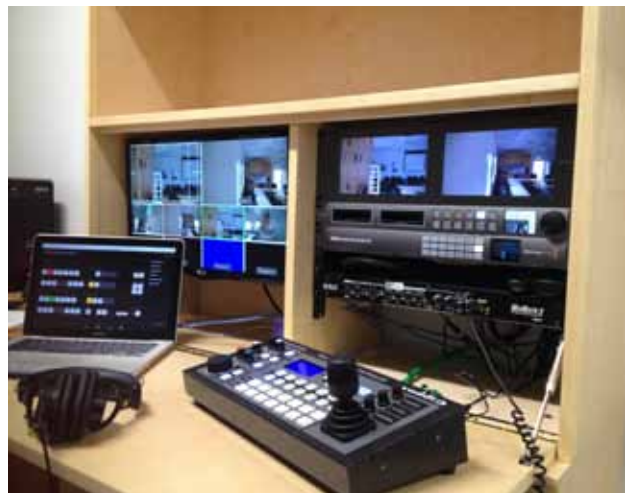
New Video Installation at Marin Clean Energy.
